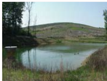
Landfill Storm Water Basin Stafford County, VA
