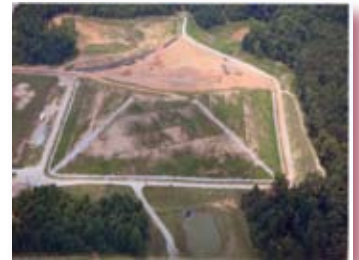
Landfill Closure Prince Edward County, VA
