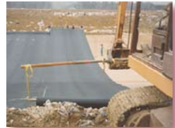
Membrane Liner Installation King William County, VA
