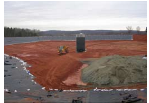
Town of Orange - Raw Water Storage Basin Outlet Structure
