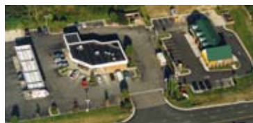
Atlee Station Hanover County, VA
