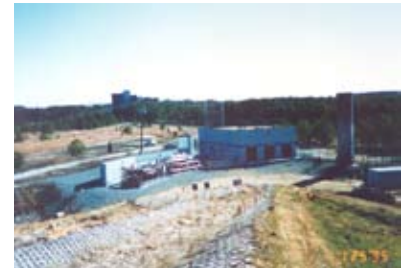
Landfill Gas to Energy
