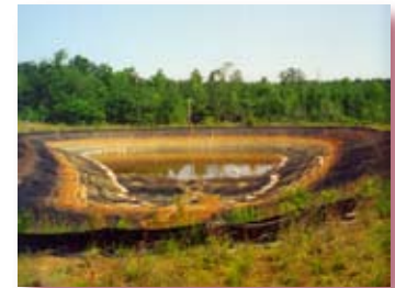
Leachate Pond Prince Edward County, VA
