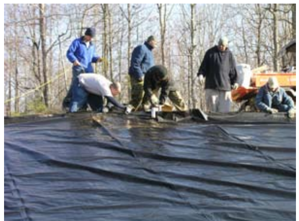
R-Board - Rain Cap Installation
