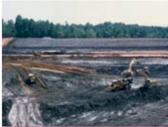
Lining Subgrade King & Queen Landfill
