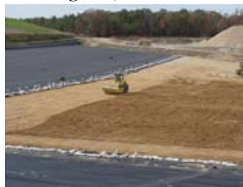
Liner Installation Ashcake Road Landfill
