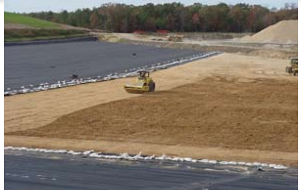
Ashcake - Liner Installation
