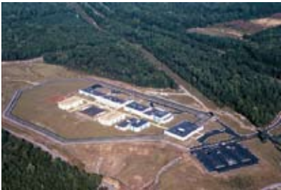
Regional Jail Facility
