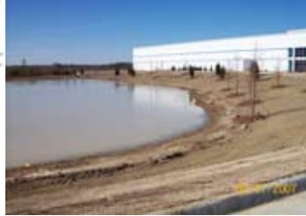
JDA Building Isle of Wight, VA
