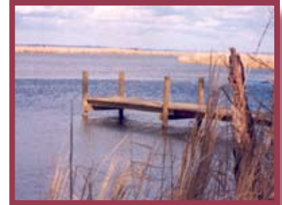
Dock Permitting (RP19)
