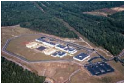
Regional Jail Facility
