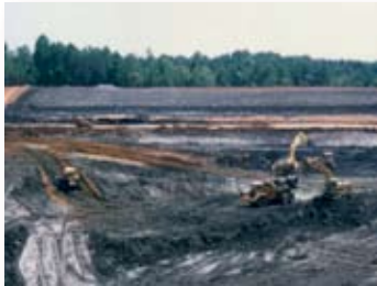
Lining Subgrade King & Queen Landfill
