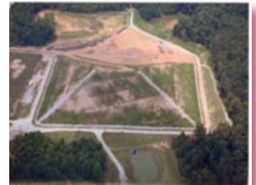
Landfill Closure Prince Edward County, VA
