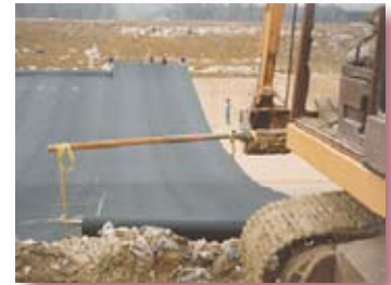
Membrane Liner Installation King William County, VA
