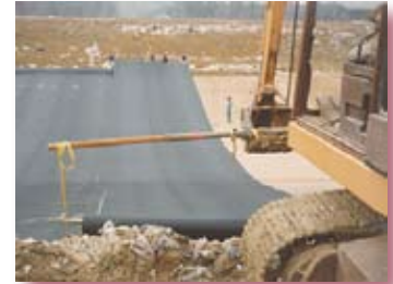
Membrane Liner Installation King William County, VA
